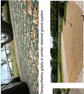
Geosynthetic geotextile or similar retained gravel system
